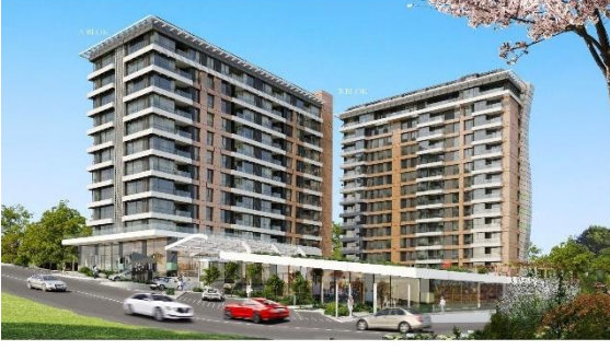
MOSTAR ATAKENT PROJESİ
